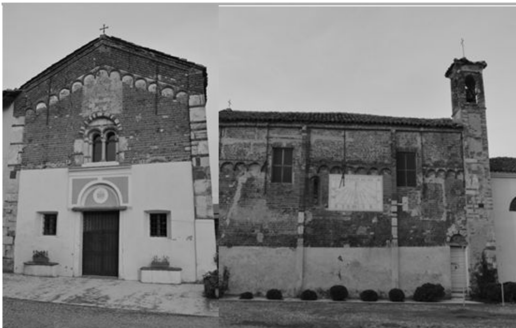
Fig. 2. Entrance and South façade of the church of Santa Maria d'Isana.
